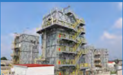
New blowout tower
