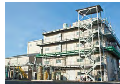
Organic iodine compound manufacturing facility
