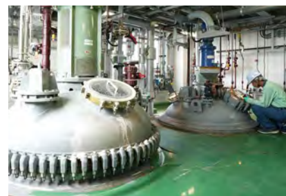
Iodate manufacturing facility
